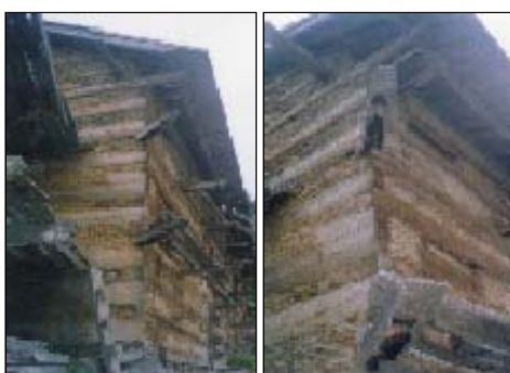
Fig. 1. Wood and stone houses—no damage due to earthquake
